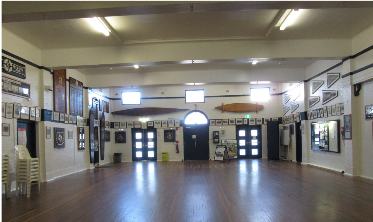
Figure 4.57: View of the central hall showing the surviving semi-circular fanlight over the front door (centre) and the three highlights above. These were originally intended to be on the sides as well but were eliminated and the, now removed, central lantern added when the design was changed to have pitched roofs on the outer side of the walls. The infilled dais is to the right. In the central bay of the ceiling, with a light on each side, is the infilled former light well / lantern location. The ceiling and beams were originally kalsomined. Source: Jean Rice Architect 2019
