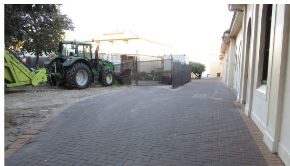
Figure 4.14: 2019 view from west of path between the two buildings showing the works yard. Source: Jean Rice Architect
