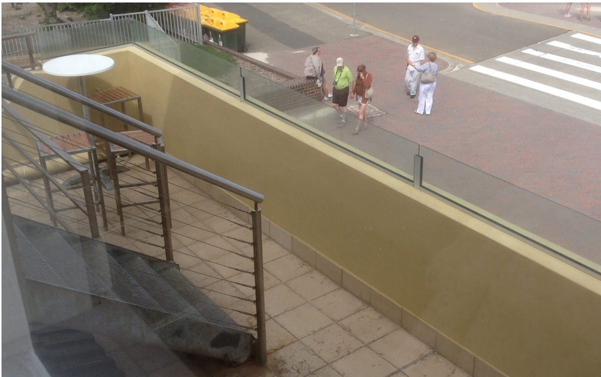
Figure 4.76: View showing the open space behind the parapet at the front. This area is at a lower level and was not originally linked to the sunbaking terrace. The highlight windows in the front wall of the hall open onto this terrace. The level of the parapet has been raised with glass panels, presumably for safety. The current stair is in a different location to that shown on the 2005 drawings but the location may have been changed during construction. Source: Jean Rice Architect
