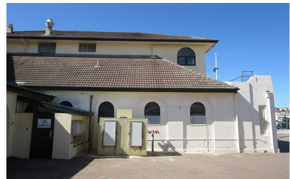
Figure 4.48: Side view adjacent the pavilion with original first floor walls, first floor additions, wet entry (at left) and free standing ice chest. Source: Jean Rice 2019
