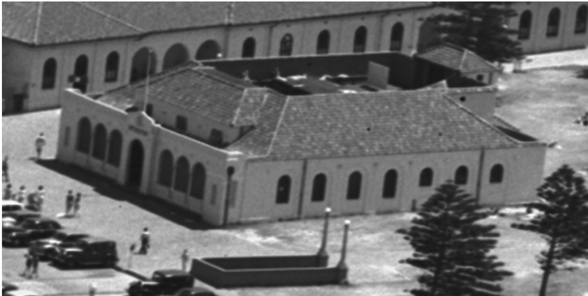
Figure 2.28: Enlargement of a late 1930s (after 1934 and before 1942) Hurley view showing the original form of the building with the roof terrace and flat roofed lantern. There are no doors on the side walls and the sill heights differ from today. The tunnel entrance is visible and the pine trees are semi mature. There is no rear compound visible and the ground is uneven grass and sand. Source: Frank Hurley NLA order
