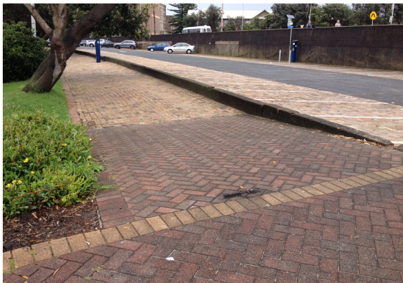
Figure 4.22: The new and old paving where the path is raised and replaced at the eastern bridge. Source: Jean Rice 2015
