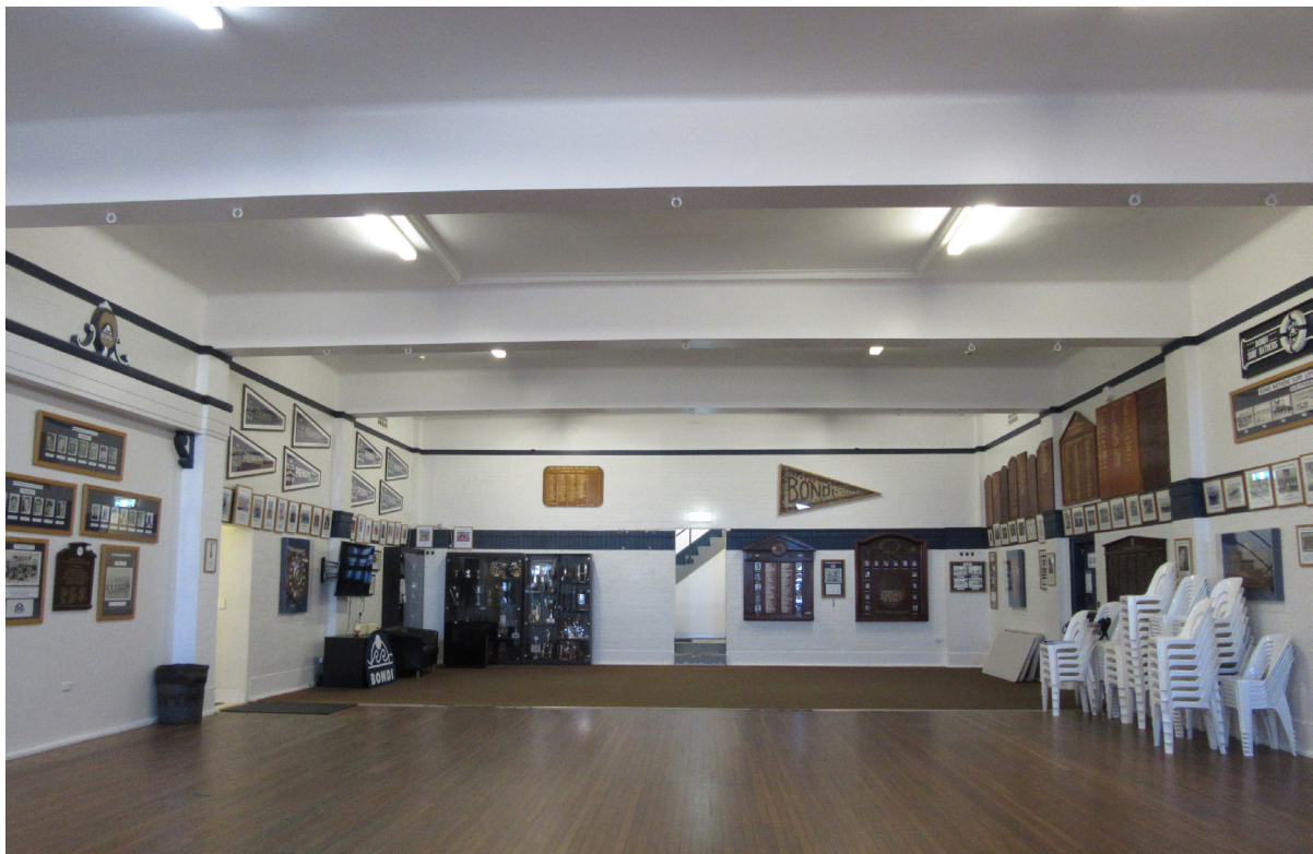
Figure 4.58: View of the central hall looking towards the back wall. The added doorway to the rear stair and corridor is in the centre of the wall. In the rear corners below the now painted brick band are the vent shafts. The infilled dais is to the left. In the central bay of the ceiling is the infilled former light well / lantern location. The metal rings for slinging boats are visible on the underside of the beams. Source: Jean Rice Architect 2019
