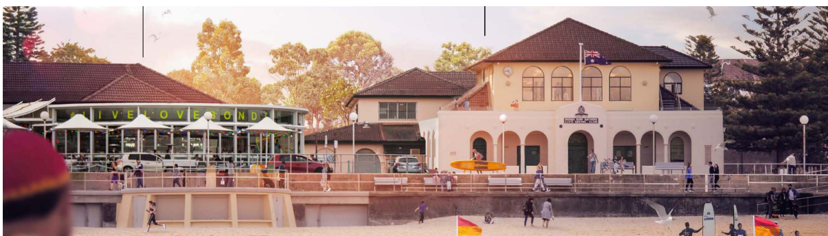
Figure 4.12: 2018 view from the water. The path between the two buildings is obstructed. Source: BSBLSC DA 2018
