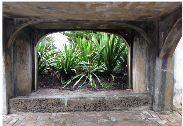
Figure 4.23: The opening under the eastern bridge now has a raised garden bed behind it. Source: Jean Rice 2015
