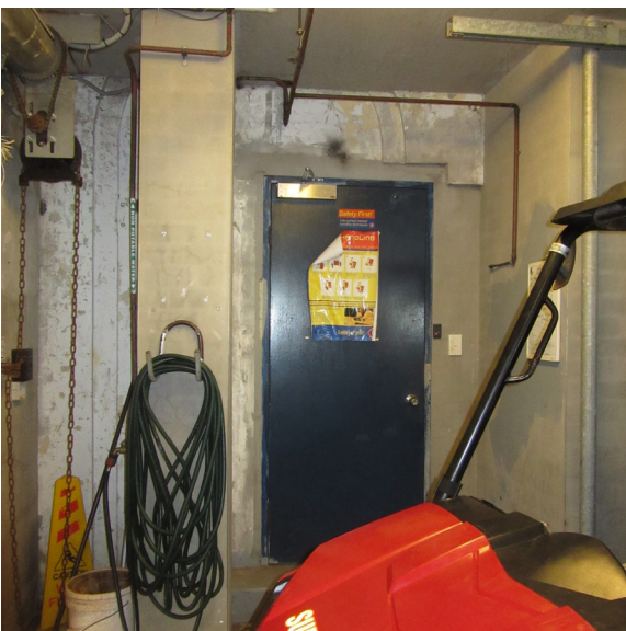
Figure 4.73: New door to corridor from boatshed. Remains of external render panel visible. Source: Jean Rice 2016
