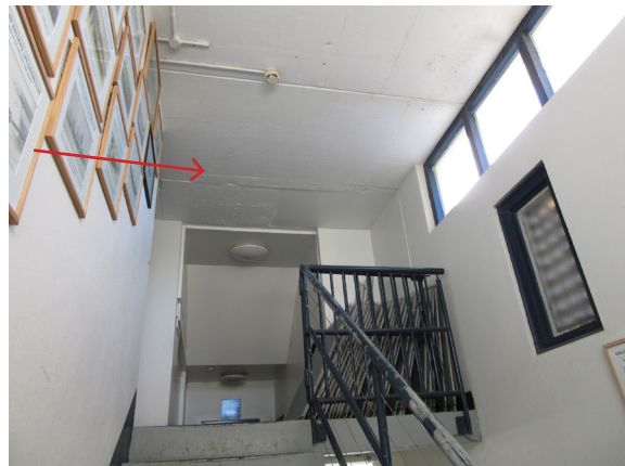
Figure 4.82: Rear stair, original vent on right with altered window over. Stair to gym across landing. Line of former shower in concrete ceiling arrowed. Source: Jean Rice 2019
