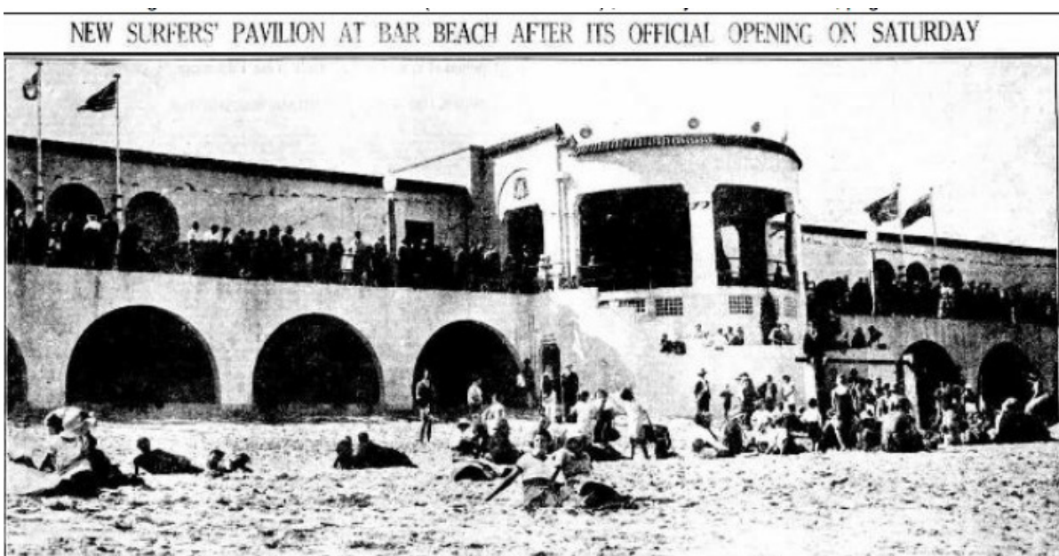
Figure 5.17: New surfer's pavilion at Bar Beach after its official opening. Source: Newcastle Morning Herald 9 October 1933
