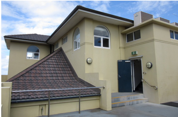
Figure 4.85: Rear terrace showing landing and entry from rear stair. Source: Jean Rice 2016
