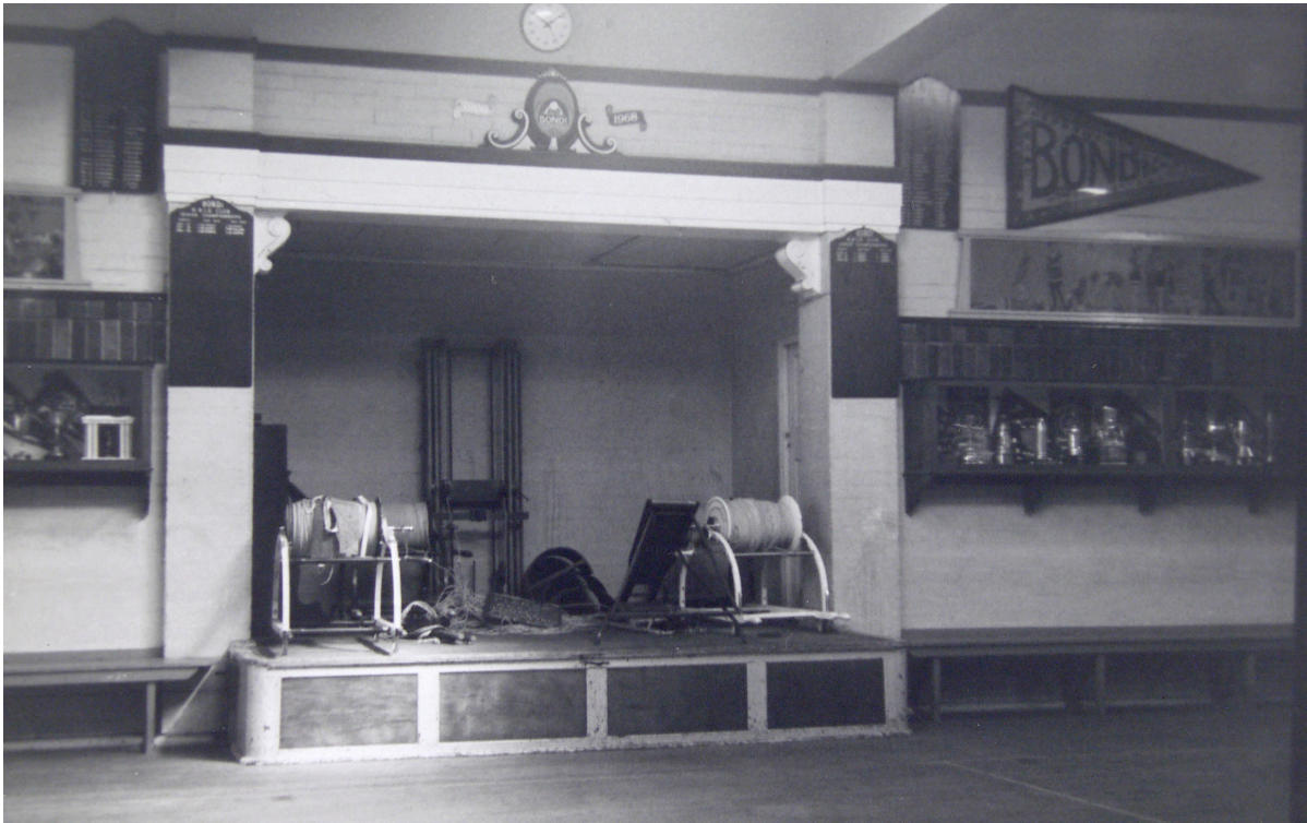
Figure 2.26: View showing the original configuration of the stage, with the mural, decorative brickwork, timber benches and trophy cabinets. Source: Digital Masters BSLSC 493
