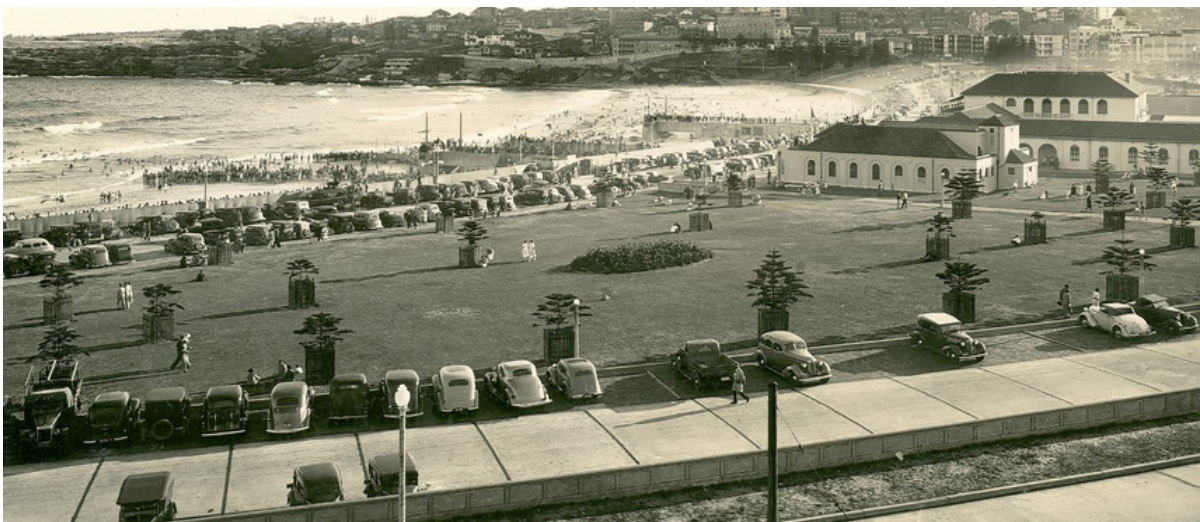
Figure 4.19: View taken between 1934 when the new club house was finished and 1942 when the groynes were removed. The pine plantings are clearly shown with timber paling tree guards and one oval garden bed. Source: SRNSW Series 12932
