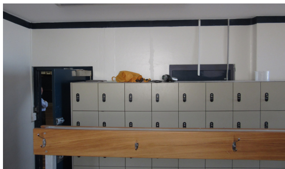
Figure 4.68: Female change room looking towards hall. Original opening with new door at left. Original closed opening behind lockers at right. Source: Jean Rice 2015
