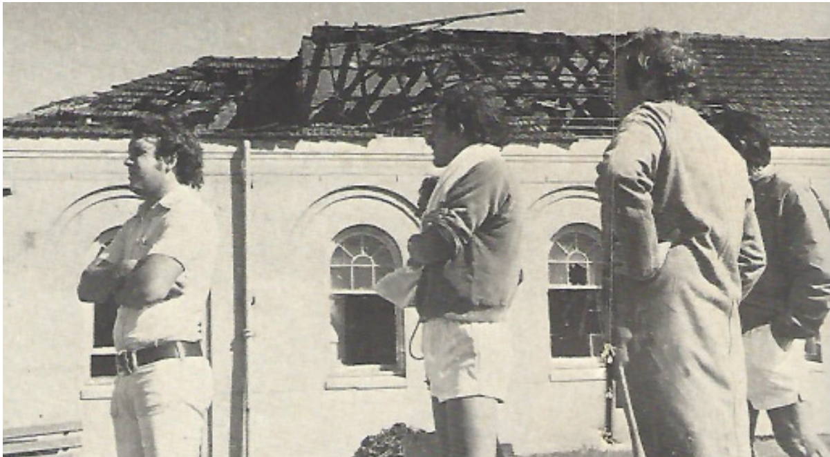
Figure 2.42: The fire-damaged club house forms a backdrop to members and inspectors checking the surf. Note the broken windows in the office area and the damaged section of roof above. Source: BSBLS AR 1973-74
