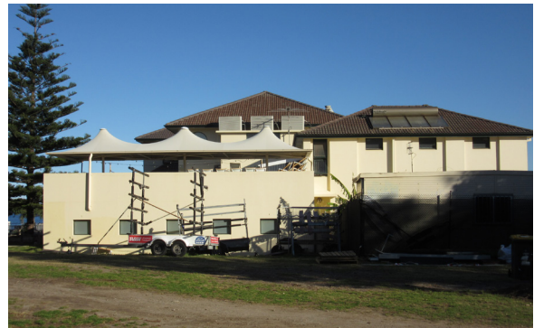
Figure 4.44: The rear of the building with the boatshed on the left, works yard on the right and behind it the 1974 squash court addition. Source: Jean Rice 2019
