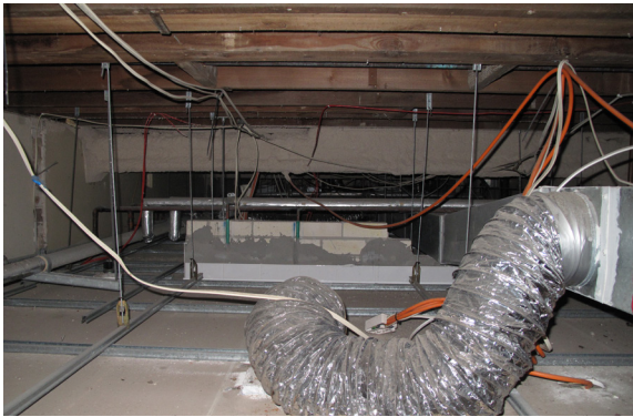
Figure 4.69: Typical - false ceiling space over female change room, masonry partition protruding. Source: Jean Rice 2015
