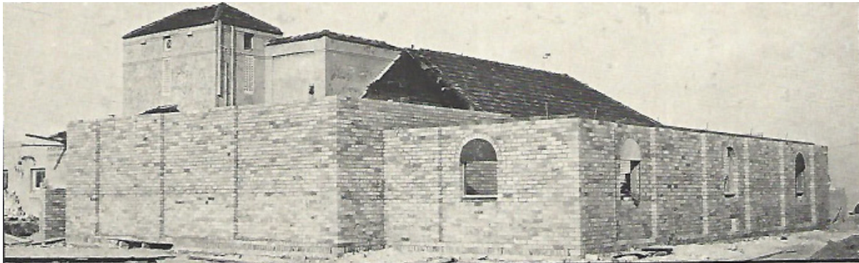
Figure 2.43: View showing the progress of the rear additions, 1974. Source: 1973-74 BSLSC AR
