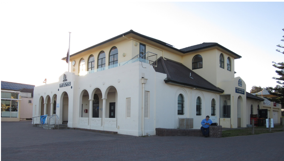
Figure 1.8: 2019 view of the Bondi Surf Bathers Life Saving Club showing the first floor addition. Source: Jean Rice Architect
