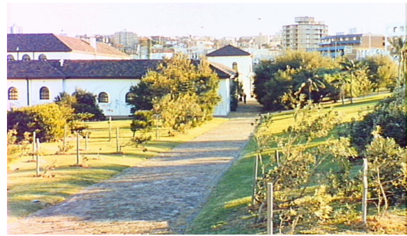
Figure 2.51: Mid 1980s photo showing original paving behind the Pavilion and more advanced plantings. On the left of the path in the foreground the plants are not thriving. Source: WC LSC WIL 304
