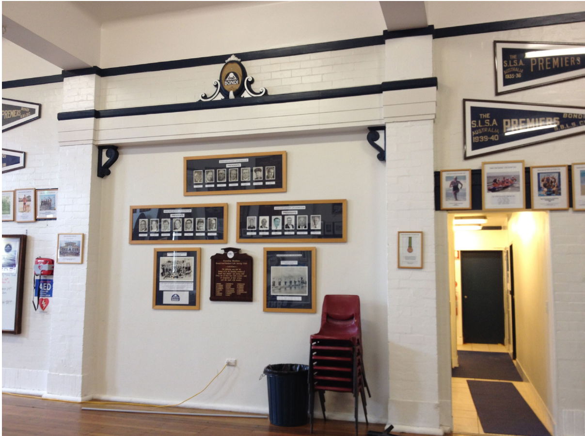
Figure 4.60: View of the infilled dais with the surf club crest over. The soldier course of bricks that forms the skirting is also visible but is painted. To the right is the entry added in 1974. Source: Jean Rice Architect
