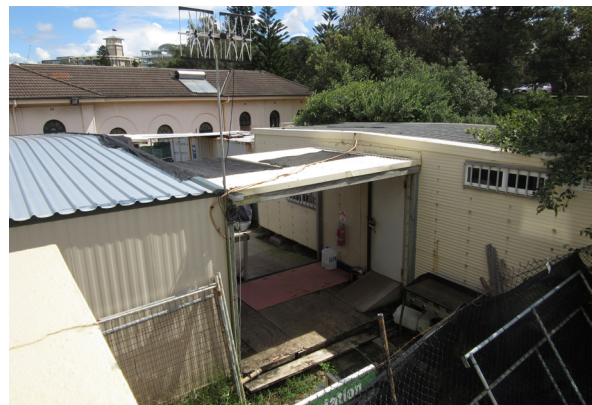
Figure 4.38: View of works yard portable buildings and covered way from the club terrace. Source: Jean Rice 2016
