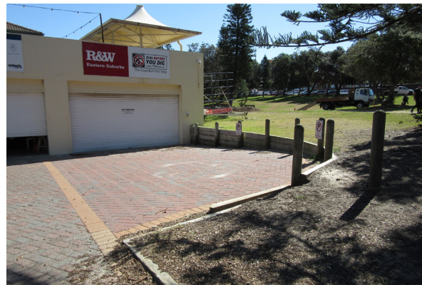
Figure 4.40: Low timber retaining wall and bollards to driveway in front of boatshed. Source: Jean Rice 2019
