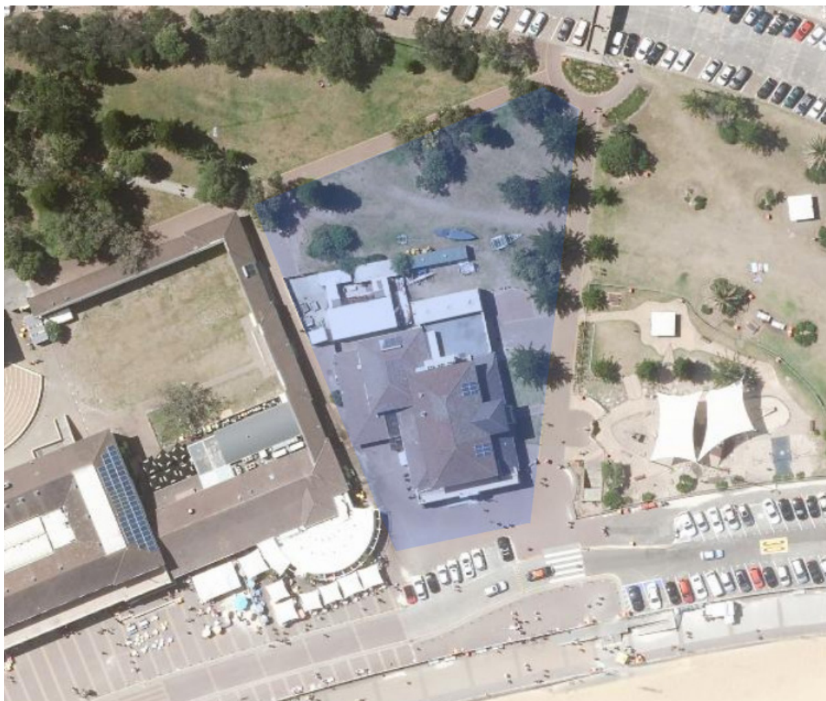
Figure I.6: c2014 aerial view of the BSBLSC with the site area for this CMP shaded in blue. The dark green shipping container behind the surf club has been removed since this photo was taken. Source: SIX Viewer, colour overlay by Jean Rice Architects
