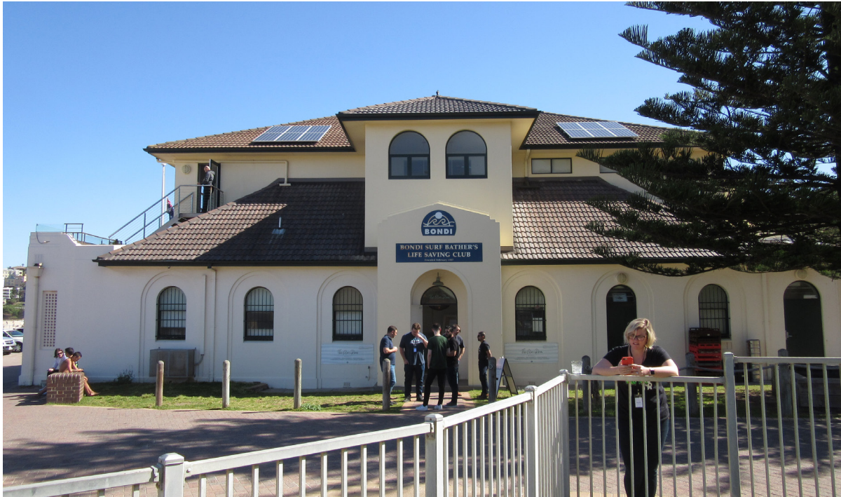
Figure I.3: 2019 view of the side entrance of the Bondi Surf Bathers Life Saving Club. Source: Jean Rice Architect
