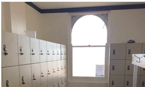
Figure 4.67: Front window of female change room. Original opening and sill height. Rectangular head to upper sash with masonry arched opening behind. Source: Jean Rice 2016
