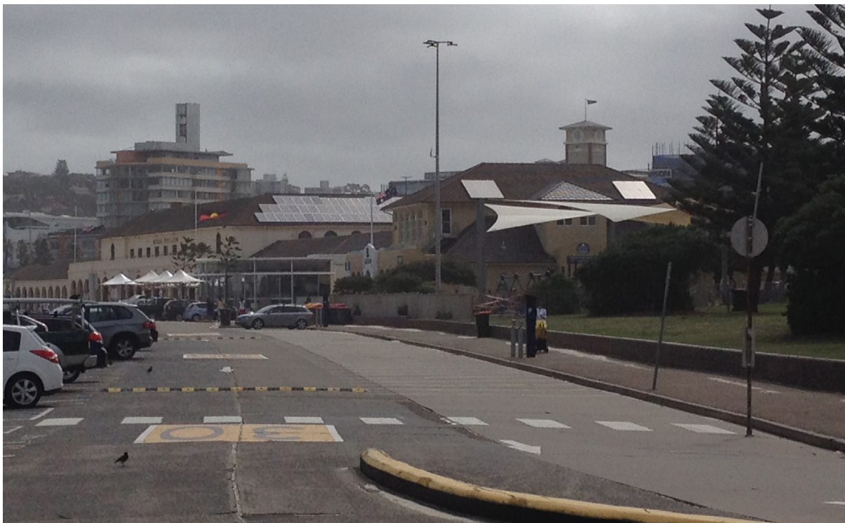
Figure 9.4: Originally this view would have featured the surf club arcade with the pavilion arcade behind. The bucket List restaurant interrupts this view and the raised ground levels, fence and plantings in the playground in front obscure the surf club arcade. Now the first floor addition dominates the club and solar panels and shade cloth intrude upon the intended views. Past views of Queen Elizabeth Drive show the main facades to have been more prominent. Note the tower of the Bondi Hotel beyond the club, which pre-dates the improvement scheme. Source: Jean Rice
