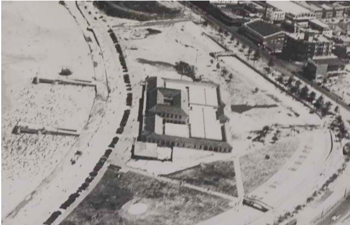
Figure 2.19: This aerial photo, probably 1928-29, shows the pavilion completed and much of the roadways and groynes. The tram loop remains at the top of the image and the old surf club remains north of the pavilion. There is a fenced compound at the rear of the club (bottom of image). Much of the park is exposed sand dunes but the area to the north has been levelled, possibly grassed, and there is a circular garden bed but no tree plantings (bottom of image). There is a diagonal line behind the club house and pavilion - possibly the edge of the construction site Source: AA
