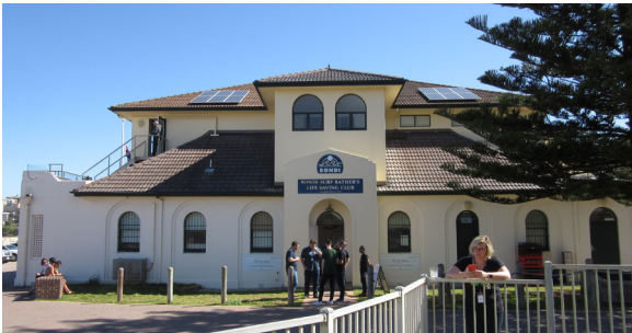
Figure 4.45: Side view showing the 2005 entry and stair to the first floor function room with the porch designed to match the original at the front. Source: Jean Rice 2019
