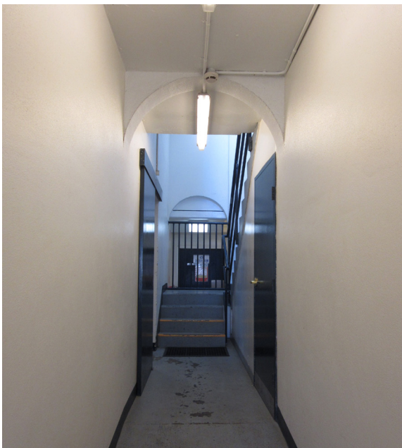
Figure 4.71: Rear corridor looking south. New stair blocks former access. Source: Jean Rice 2019
