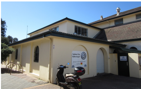
Figure 4.47: Side view adjacent the pavilion of the 1974 rear and first floor addition. The roller door is to the IRB store Source: Jean Rice 2019
