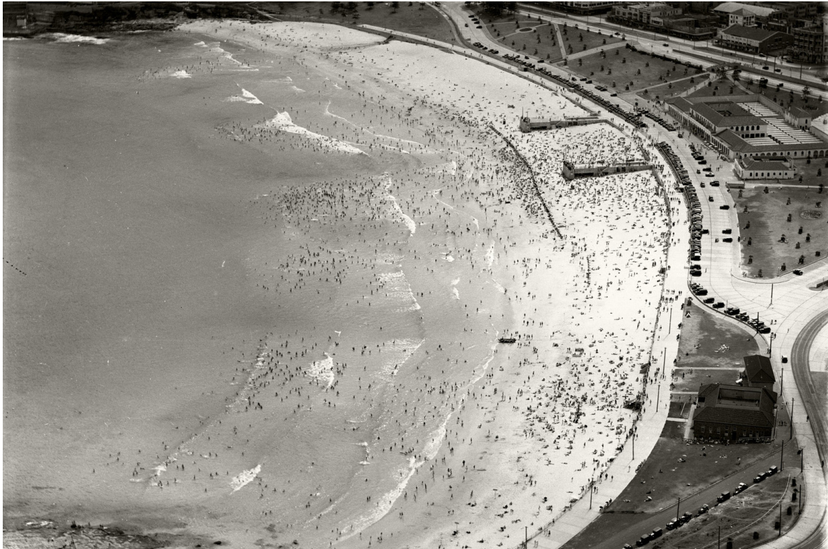
Figure 2.31: 1937 aerial showing the surf clubs erected in 1934 (right centre and bottom right), both of which had a rooftop sunbaking area and an observation deck. Source: Adastra (via RAHS)
